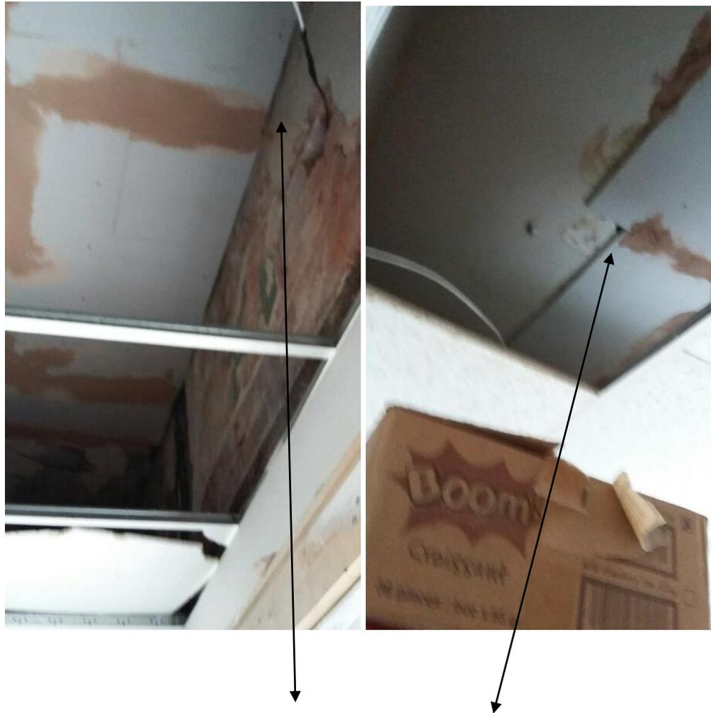
Picture above show gaps and holes to the fire separation between floors, which can only be maintained by adequate fire boarding that has been properly filled or plaster board with a layer of skim plaster finish.
